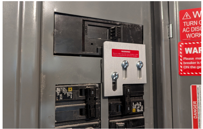
Mechanical interlock to toggle between grid and backup power
