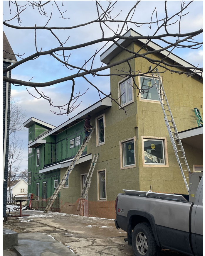
Rockwool Installation
